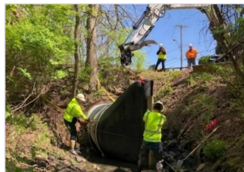
USACE Buffalo District contractors install a check valve at Wolf Creek in Barberton, Ohio, on May 13, 2020, as part of the Ohio-Erie Canal Aquatic Nuisance Species Barrier Project in Akron, Ohio. (Credit: Andrew Kornacki)
