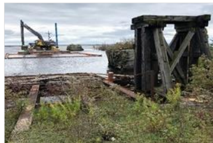
Mechanical dredging of PCB-contaminated sediment from a barge on the river. (Credit: Julie Simmons, NOAA)
