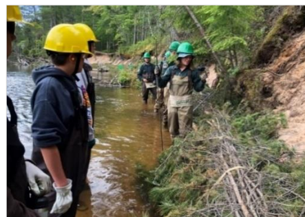
Installing and inspecting readily available materials recently used to stabilize eroding streambanks in the Au Train River. (Credit: USFS)
