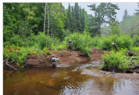
Crews work to stabilize streambanks on the Pilgrim River. (Credit: Sustainable Research Institute)
