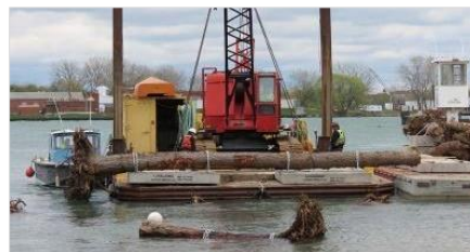
Placing log structures along the shore to deflect wave energy. (Credit: New York State Department of Environmental Conservation)
