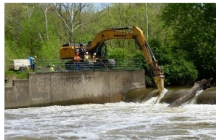
“Notching” the dam on the first day of deconstruction. (Credit: NPS)
