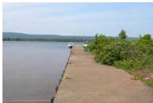
Isle Royale National Park, Lake Superior; the concrete dock and breakwall are being removed to restore habitat and enable natural sediment migration.
