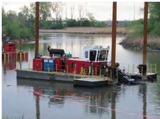
EPA is removing contaminated sediment from the bottom of the Ottawa River, located in the Maumee River AOC (Toledo, OH). This project was funded with pre-GLRI funds, but the GLRI will enable additional projects that will remove contaminated sediment.
