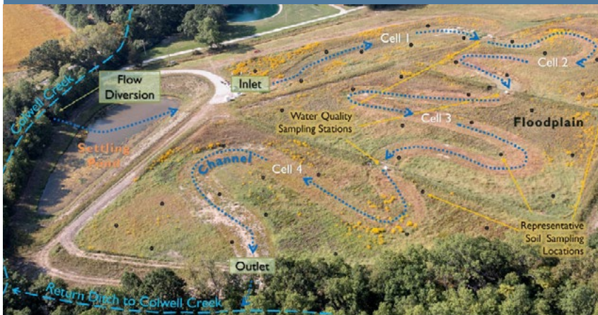
Aerial image of phosphorus optimal constructed wetland in Defiance, Ohio. Photo credit: USACE
