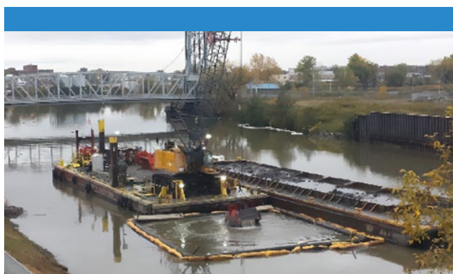
Mechanical dredging of contaminated sediment in the Buffalo River. Photo credit: Brian Murphy
