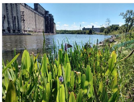
Northeastern shoreline of the Katherine Street peninsula on the Buffalo River after habitat restoration. (Credit: USACE)
