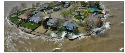
Multiple record high-water levels were set on the Great Lakes in 2019 and 2020, resulting in increased risks from erosion and coastal flooding. (Credit: USACE)
