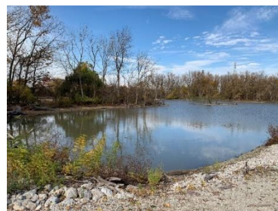
The nursery habitat embayment constructed in the northern portion of the Penn 7 habitat restoration site. (Credit: NOAA)
