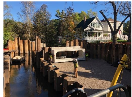
Culvert replacement underway on Kids Creek. (Credit: Zach Cole)
