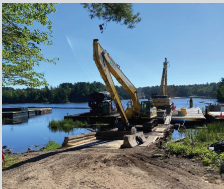
Placement of sediment cap containing pelletized activated carbon mixed with sand to absorb and immobilize contaminants in Scanlon Reservoir, Minnesota. Photo Credit: US. Army Corps of Engineers
